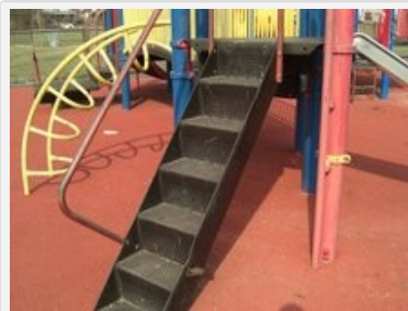
Missing handrail up to slide at Philadelphia's American Legion playground
