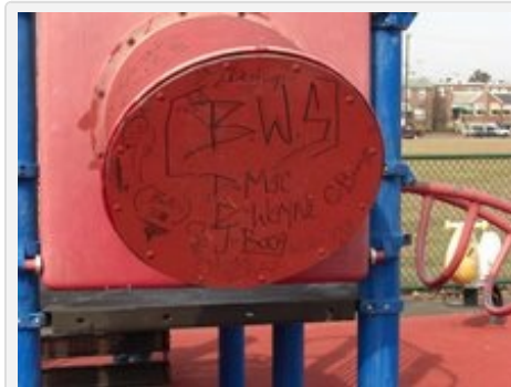
Outside view of boarded-up hole at Philadelphia's American Legion playground. Leach fears the board could collapse and a child could get hurt.
